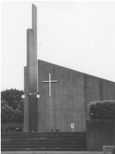
Yokohama campus chapel
