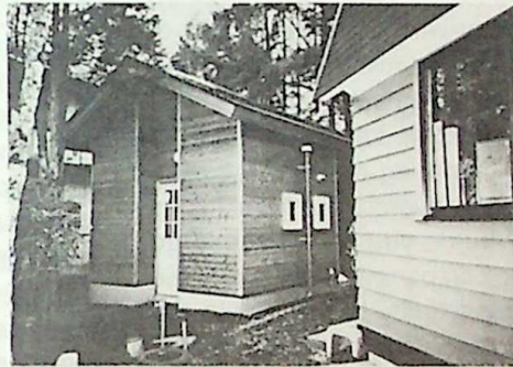
New toilet facilities
