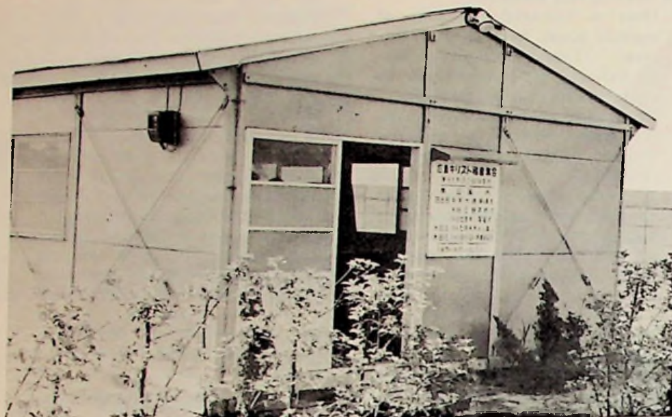
Front entrance, showing bulletin board which is lighted at night.
