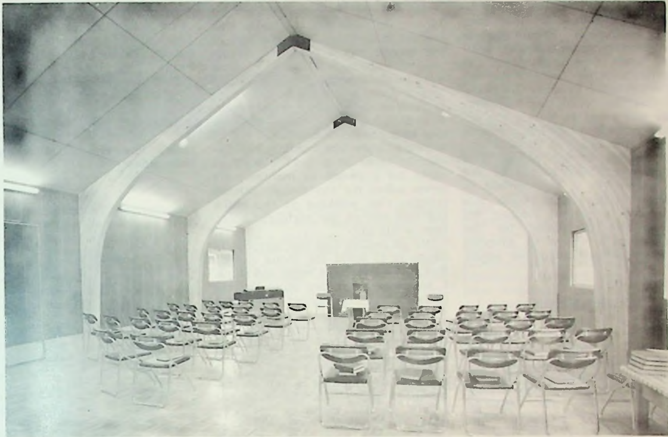
The laminated arches are effectively shown in this picture
