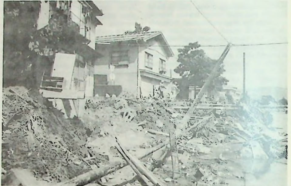
A portion of the washed-out bank of the Kamo River
