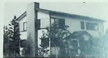
Kyoritsu Memorial Hall completed June, 1979
