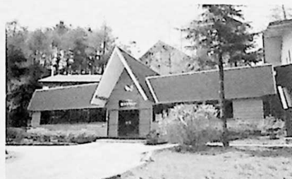
▲Newly Constructed Office & Giftshop
