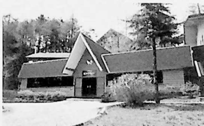
▲Newly Constructed Office & Giftshop
