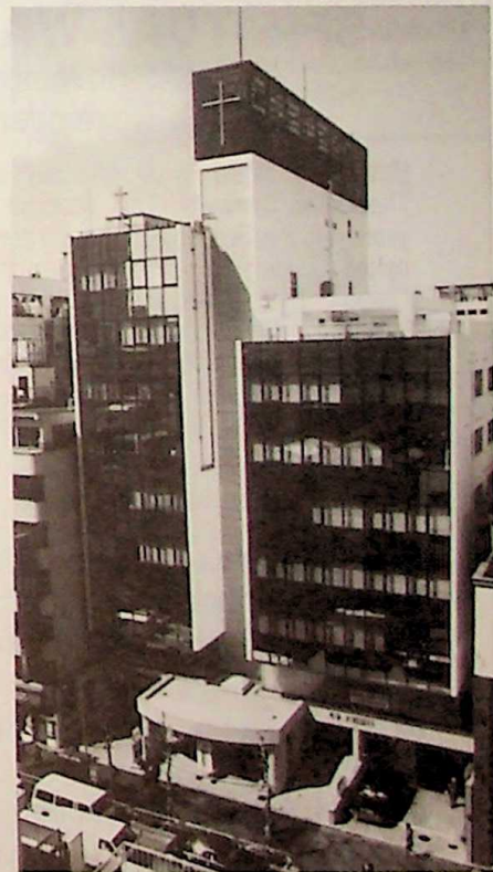
Ochanomizu Christian Center Building, home of OBI
